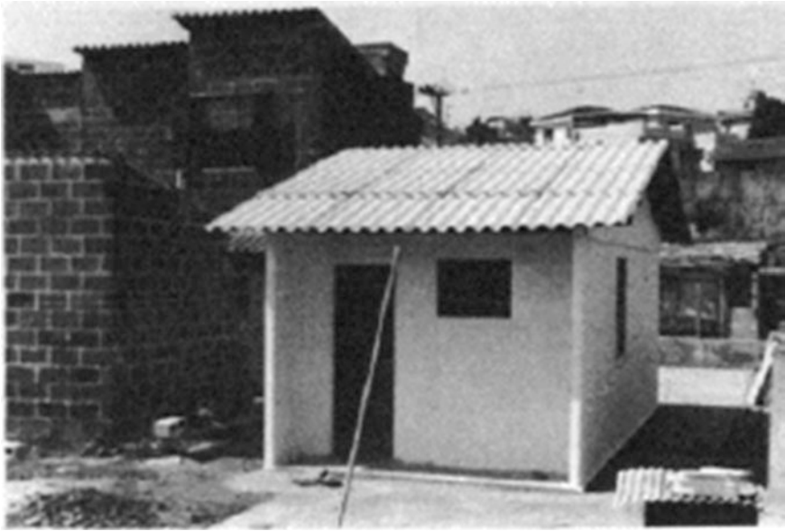
Fig. 13.11 Wall panels of affordable house made by mortar reinforced by coconut fibres (John et al. 1990)
